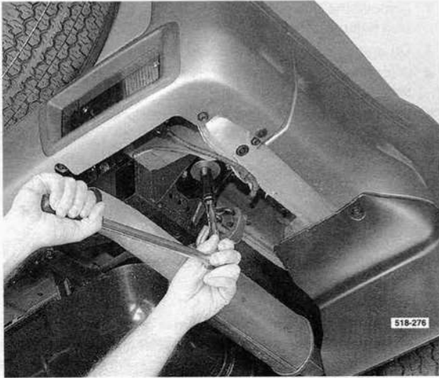
Checking that the chassis to body retaining bolts are tight.
