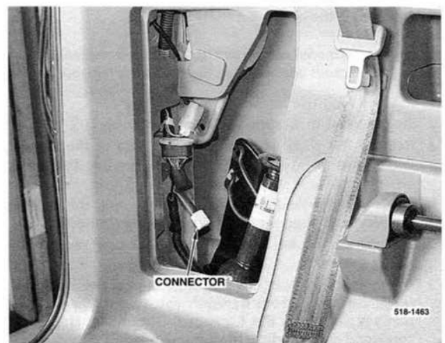
The trailer wiring connector is located in the rear quarter panel compartment.
