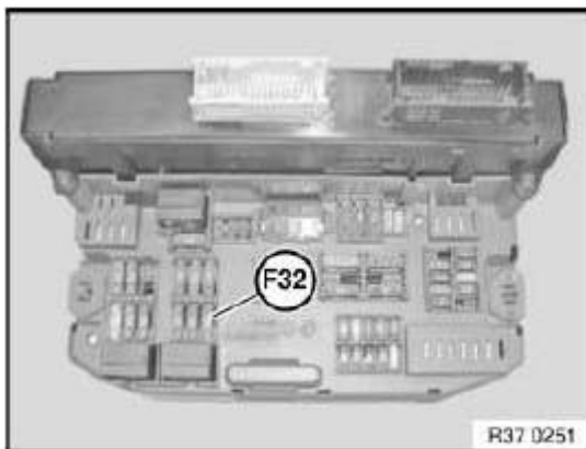
Fig. 10: Identifying Fuse (F32) Courtesy of BMW OF NORTH AMERICA, INC.
