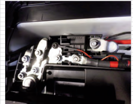
Central fuse protection at positive terminal
