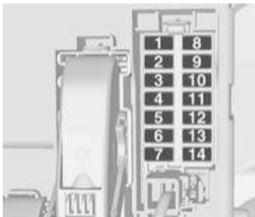
Opel Tigua Twin Top (2009) – fuse box – instrument panel
